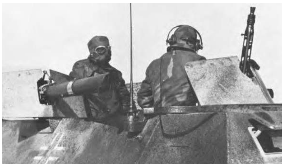
Right: This Ausf D features the later-style flame gun shields. There are larger with a smaller aperture and provided increased protection to the gunners.
