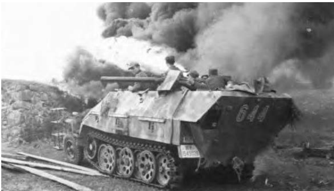
This shot of an Sd.Kfz 251/16 Ausf D taken during a demonstration shows the side-mounted flame gun to good effect. The right side gun is in operation, sending out a jet of flame. Note that the crew are not wearing the protective overalls and hoods—unpopular items that were rarely used.
