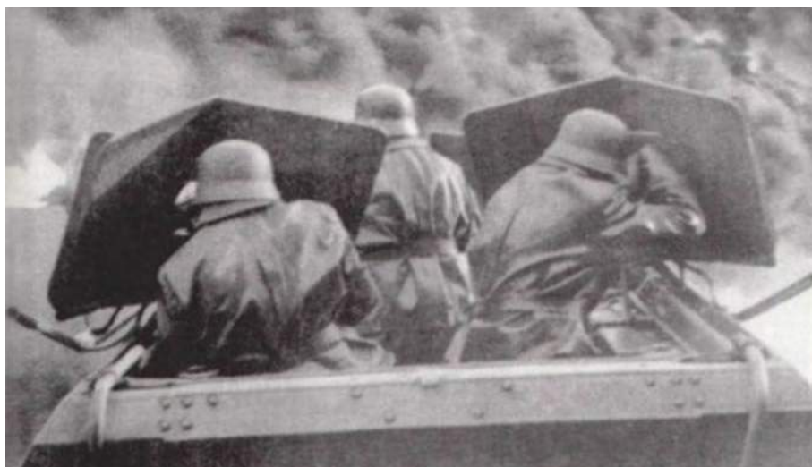
Right: This Ausf D features the later-style flame gun shields. There are larger with a smaller aperture and provided increased protection to the gunners.
