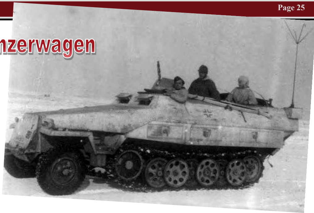
An interesting photo of a 251/3 Ausf D. Note the worn winter whitewash. Hoops for the fighting compartment cover are in place, but the cover is not. Note the skis tied to the side of the vehicle and the prominent 2 meter star antenna. Visible crewmen wear the reversible winter parka and a variety of headgear.
